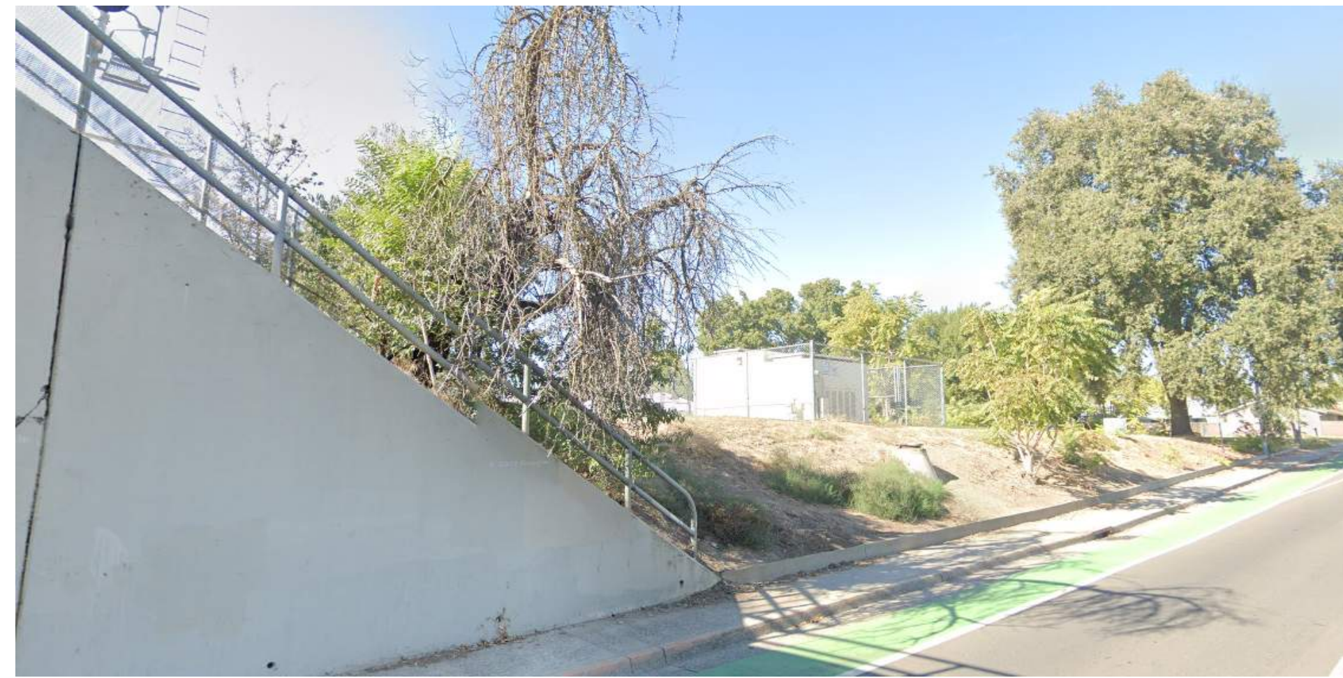
3- SOUTH VIEW FROM 5TH STREET UNDER BRIDGE
