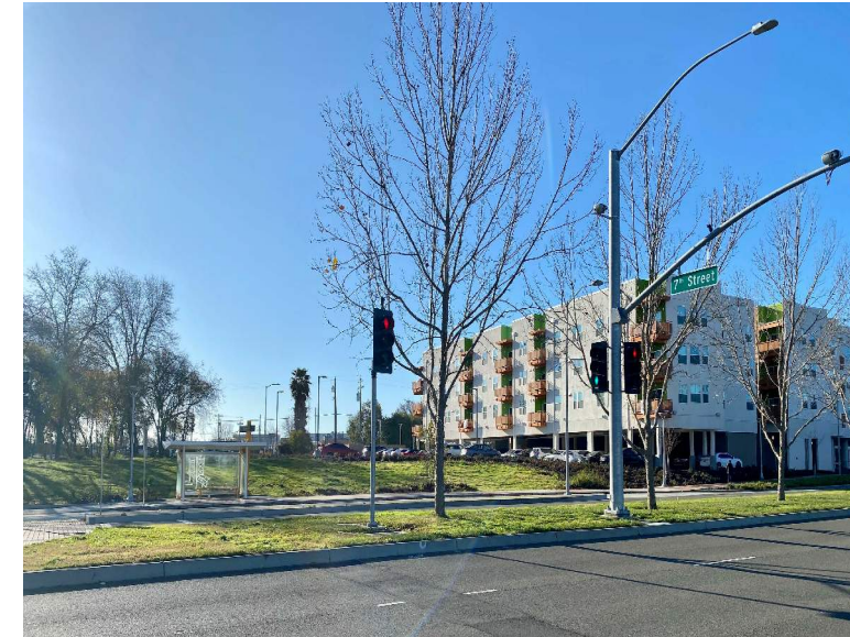
3. LOOKING SOUTH FROM TOWER BRIDGE GATEWAY AT NORTH SIDE OF SITE
