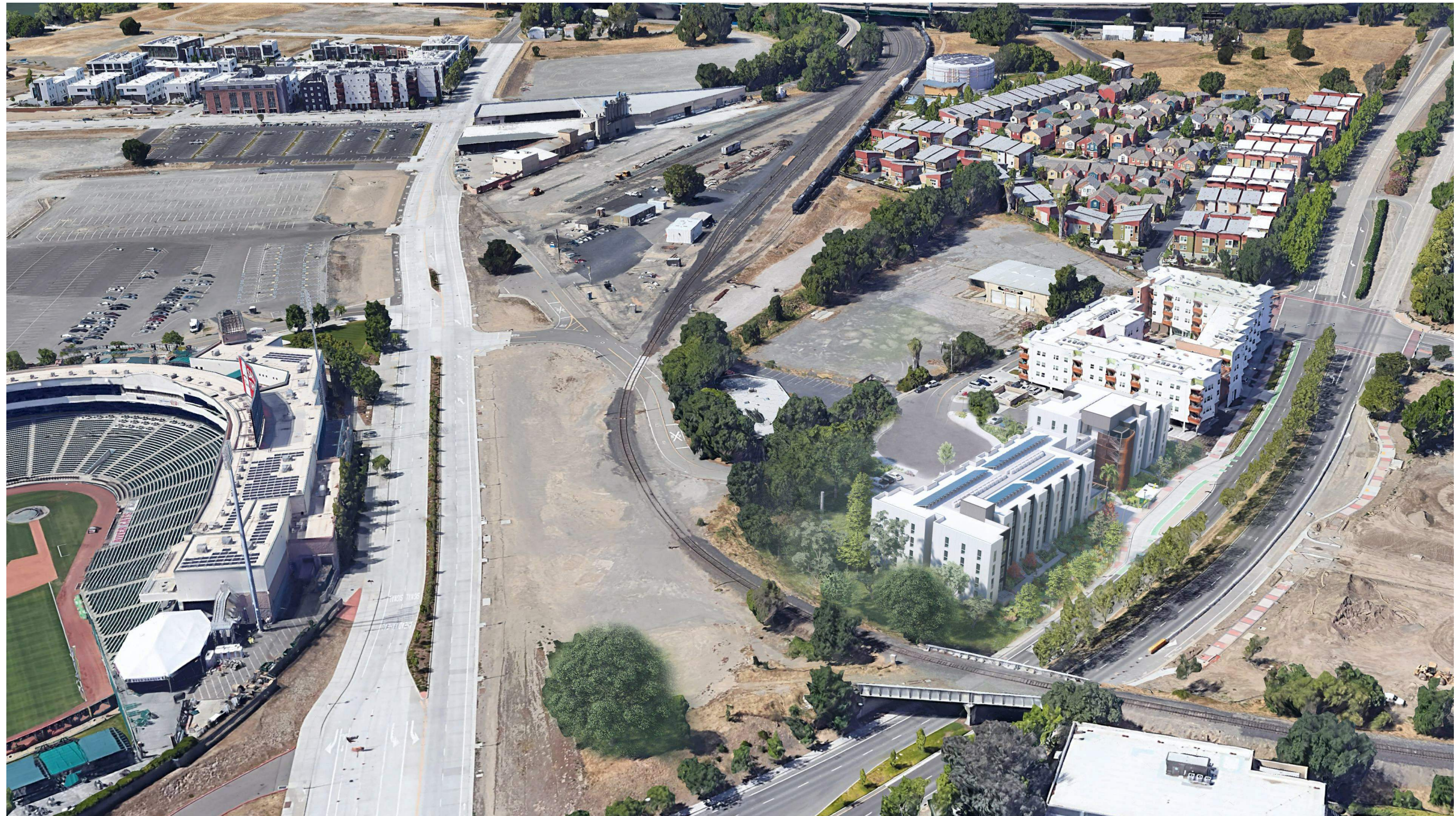
AERIAL VIEW LOOKING SOUTHWEST
